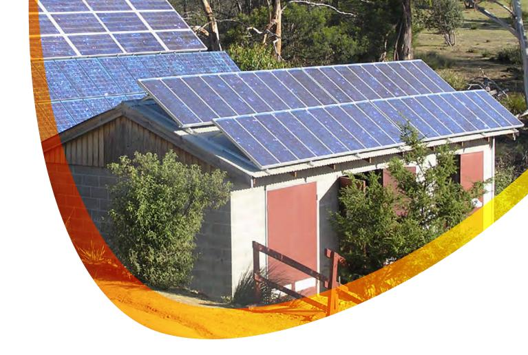
**Sunlight and panel placement** - Assess sunlight availability, considering shading from structures or trees and your area's climate. Our specialists will identify the best location, orientation, and tilt for solar panels to optimise efficiency. If your roof is small, consider a free-standing/ground mount array.
